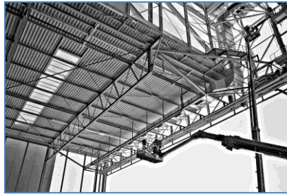
Gate air system, Airbus-Hangar
